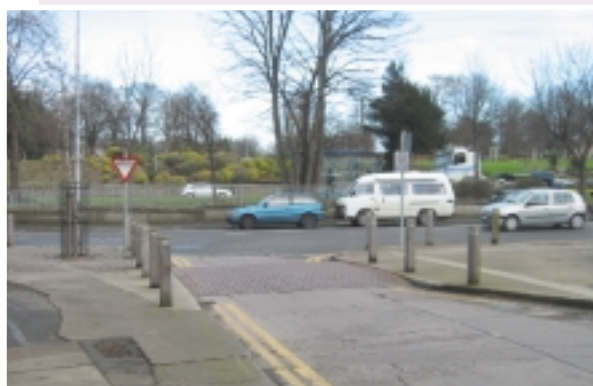
Entry treatment into an Access road
